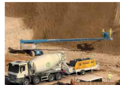
Concrete & Mortar Pump Hire
